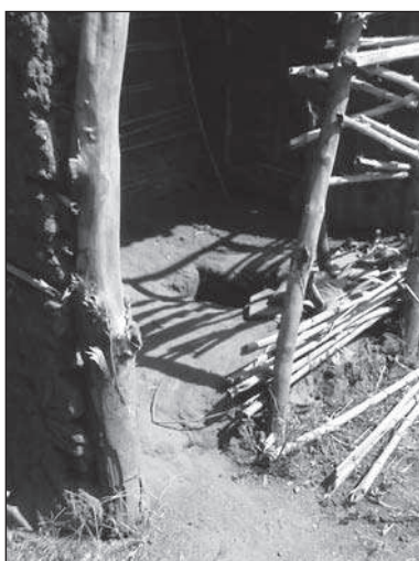
Figure 9.132. The packed earth floor of the pit latrine.
