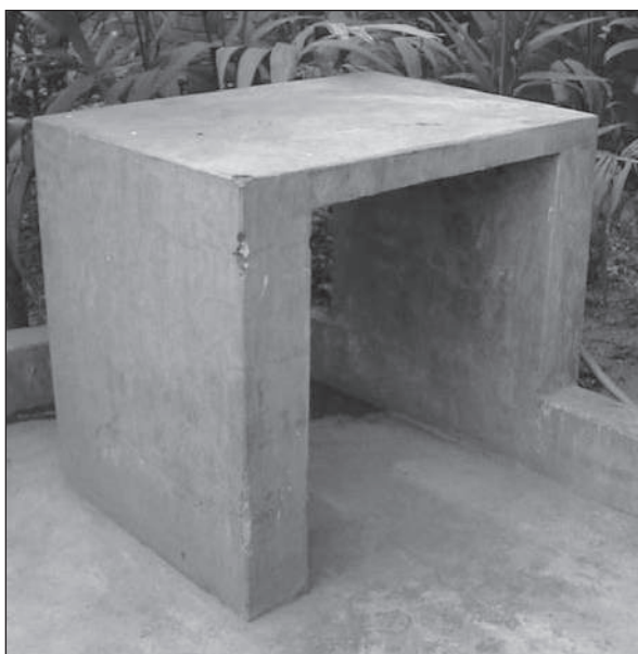
Figure 6.83. Concrete slab for washing clothes. (Case-study 9.3, page 166)
