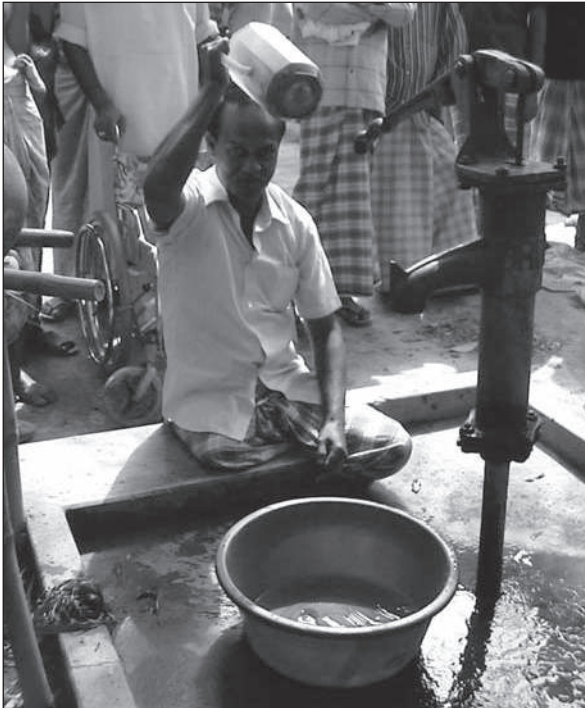
Figure 6.48. Low concrete sitting platform. (Case-study 9.2, page 161)
