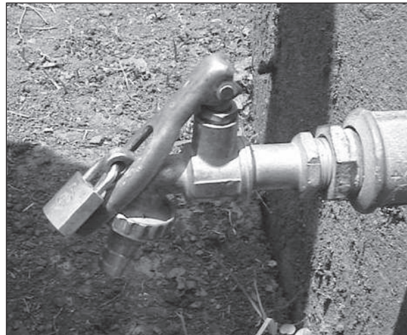
Figure 6.22. Lever operated tap with padlock. Unsuitable for a person with limited grip or stiff fingers. (Case-study 9.21, page 219)
