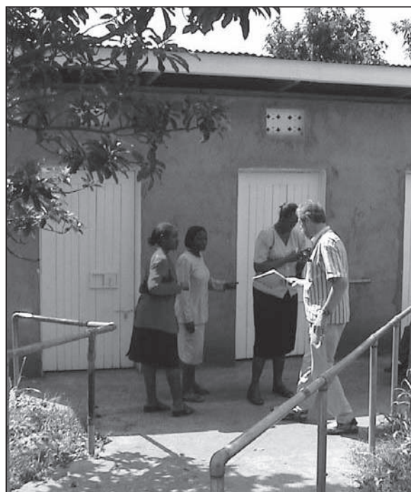
Figure 5.10. Wide concrete ramp with handrails both sides.
