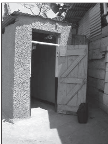
Figure 9.118. Door with a two-way hinge.
