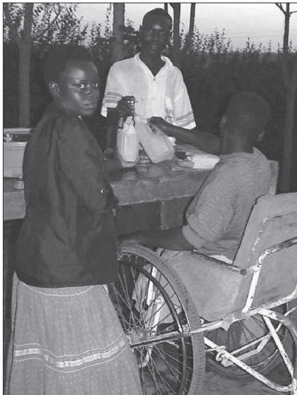
Figure 6.18. A user parks his wheelchair with his knees under the concrete shelf of a tapstand. (Case-study 9.20, page 217)
