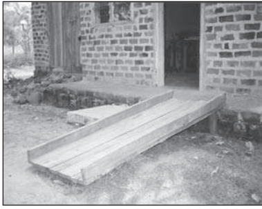
Figure 9.149. Movable wooden ramp.
