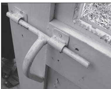
Figure 9.123. Large slide bolt for easy grip.
