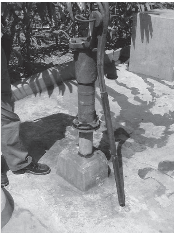
Figure 6.4. Handpump with apron showing direction of water drainage away from pump. Note lengthened handle for extra leverage.
