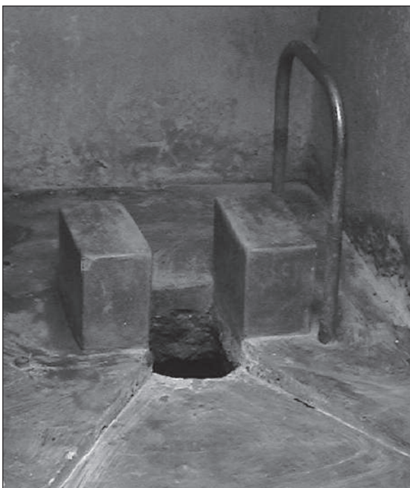
Figure 7.26. Twin cement-plastered brick sitting blocks. Height: 25cm; gap: 14cm. The gap makes anal cleansing easier than on an ordinary seat. (Case-study 9.26, page 232)
