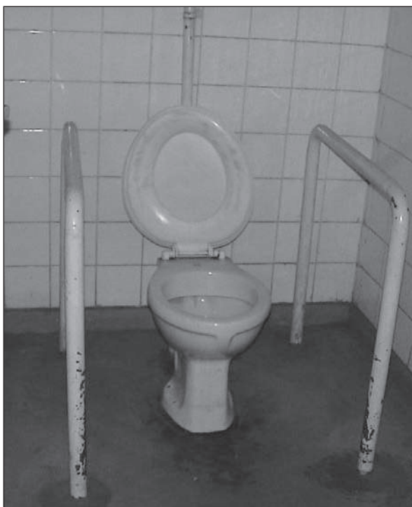
Figure 7.2. Painted handrails cemented to floor on both sides of pedestal toilet. 50mm Ø g.i. pipe; H: ~80cm.
