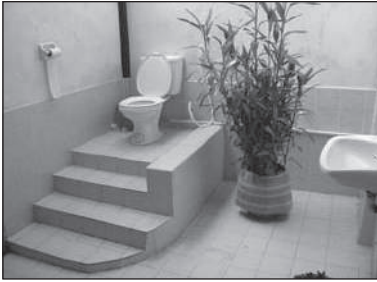
Figure 2.5. Steps to the toilet.
