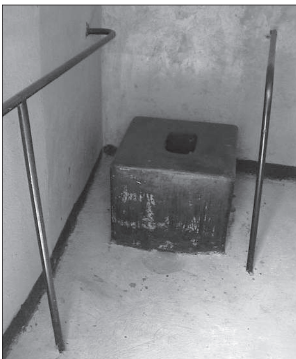
Figure 7.7. Painted rail fixed to floor and walls.
