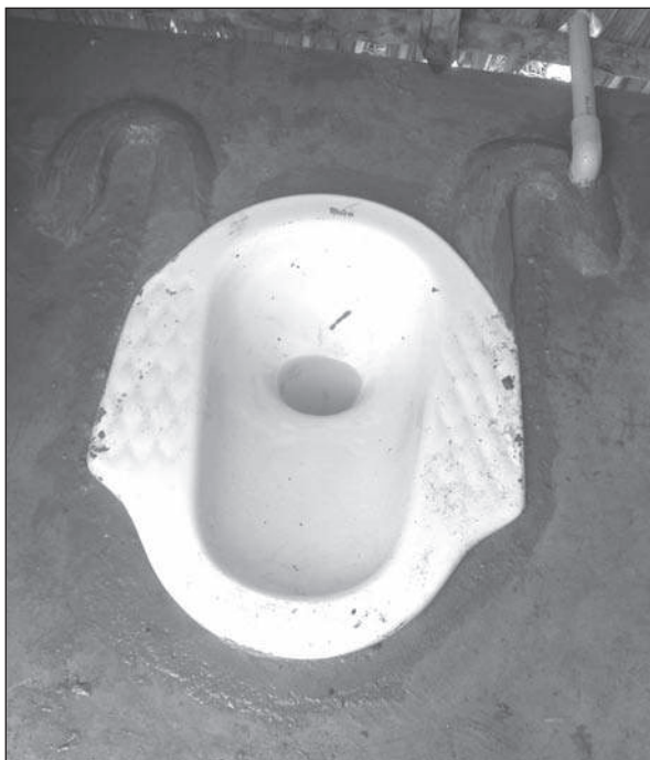
Figure 7.42. Cement mortar mouldings next to toilet pan for wheels of wheelchair to slot into for accurate positioning.
