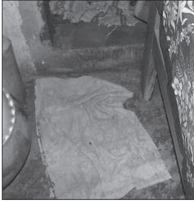
Figure 9.103 Floor cloth at the bathroom door.
