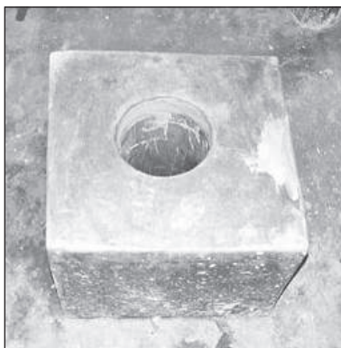
Figure 9.143. Fixed toilet seat. Note PVC pipe lining drop-hole.
