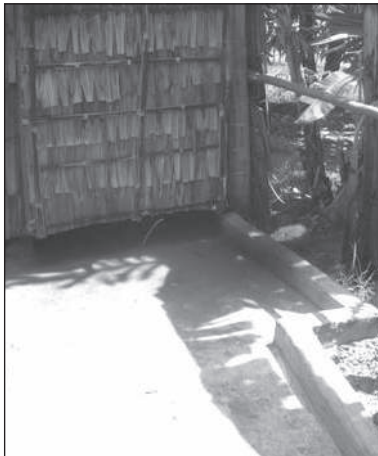
Figure 9.71. Flat platform in front of toilet door.
