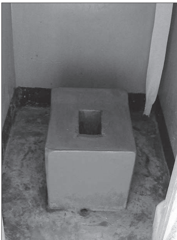
Figure 7.24. Toilet seat made of bricks, plastered with cement mortar and painted. Raised at the back for extra support. (Case-study 9.24, page 224)
