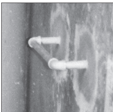
Figure 9.144. Handrail cemented to the wall.
