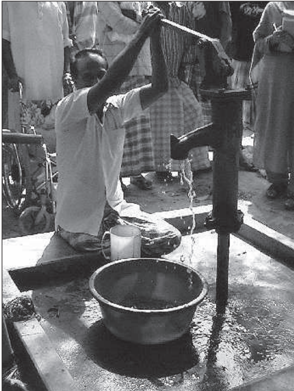
Figure 6.3. Low concrete sitting platform built into pump apron.
