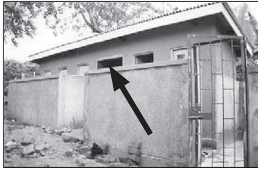
Figure 9.141. Toilet block (under construction). Arrow shows wider doorway of accessible toilet in the centre.
