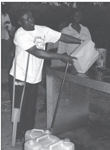
Figure 9.98. Raised tapstand with shelf to rest containers on.
