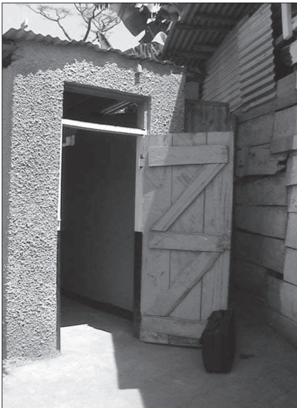
Figure 5.20. Toilet door with a two-way hinge allows this door to open outwards and inwards. Note the international disability symbol on the door.
