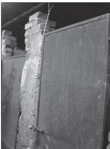
Figure 9.40. Rope hanging from roof beam.
