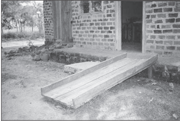
Figure 5.12. Movable wooden ramp.
